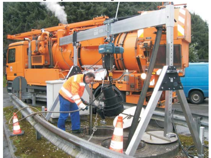
Maintenance work on a dirty water pump
